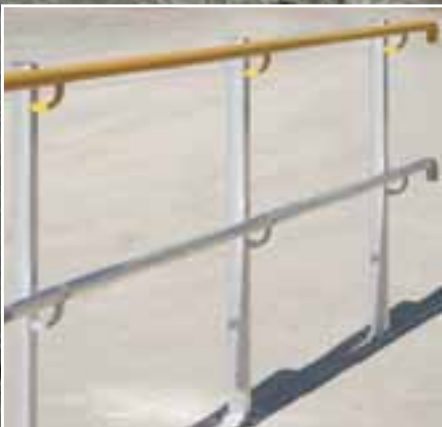
for a DDA compliant handrail
