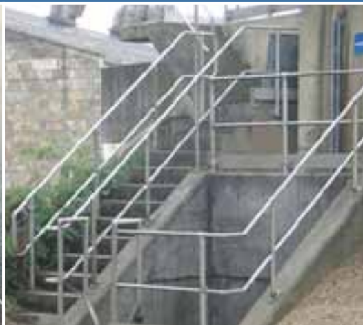
Tadcaster Water Treatment Works
