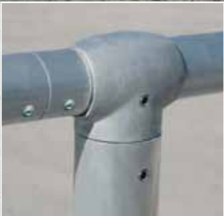
mechanical fixings to all connections
