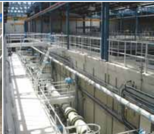
Headingley Water Treatment Works
