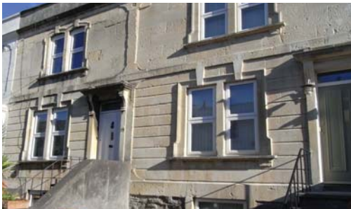
Top left: Mixed use of PVC-u and wooden windows in the same elevation
