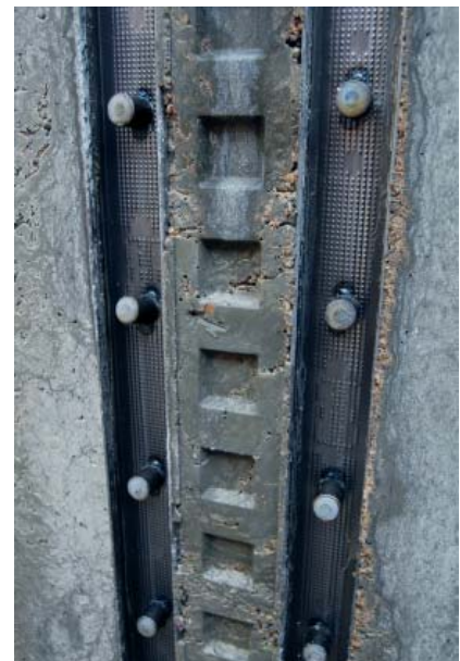
Concreting result: position of the Coupler sleeves within the indented joint
