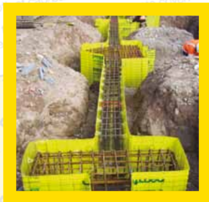
Check concrete cover. Fix Pecafil spacers.
