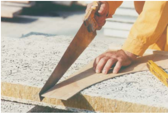
Cutting with handsaw
