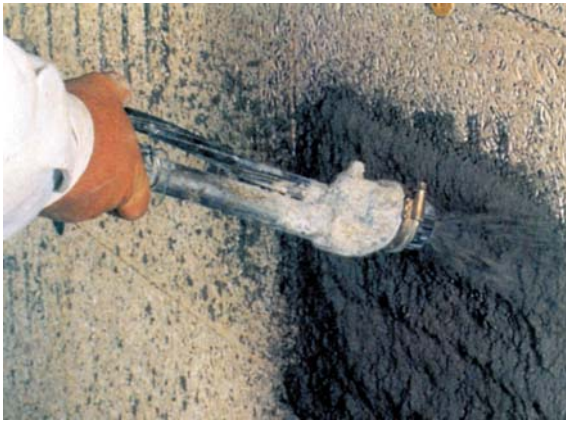
Applying the plaster undercoat
