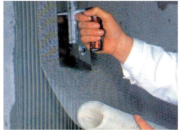
Applying the reinforcement layer
