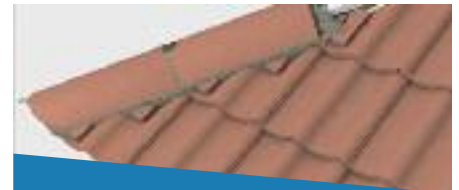
Mortar bedded security hip
