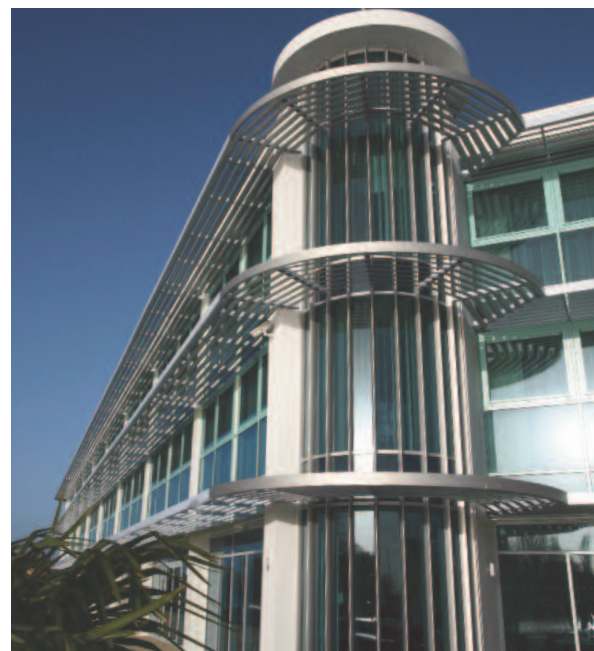
The Captain's Club Hotel in Poole benefits from the flexible and aesthetically pleasing Levolux Matrix XL Solar Shading System.
