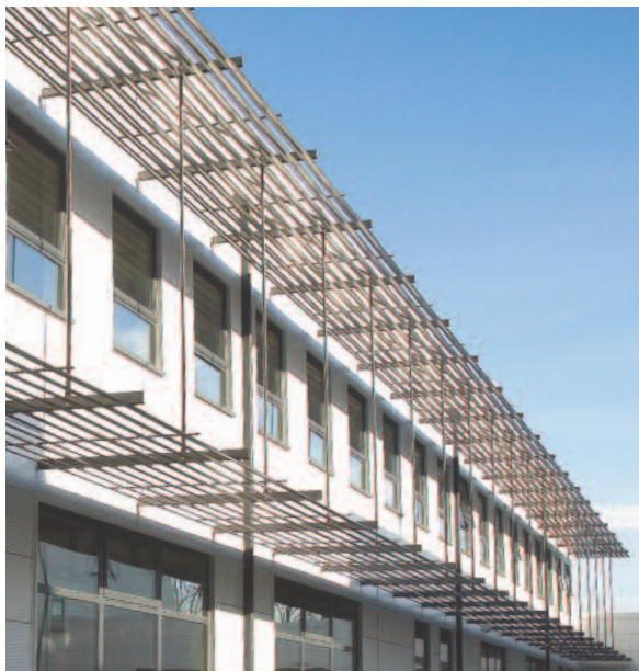
Levolux installed its striking Matrix XL system, with 'Z' section louvres above each row of windows at Haringey 6th Form College.
