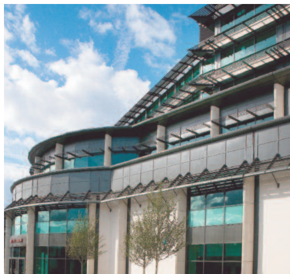
The new South Stand of the RFU Twickenham Stadium in Middlesex is fitted with the Matrix XL Solar Shading System with an integral Walk-On Platform.
