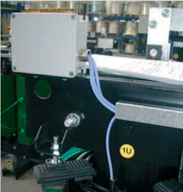
Example of installation of a Pt100 temperature control unit
