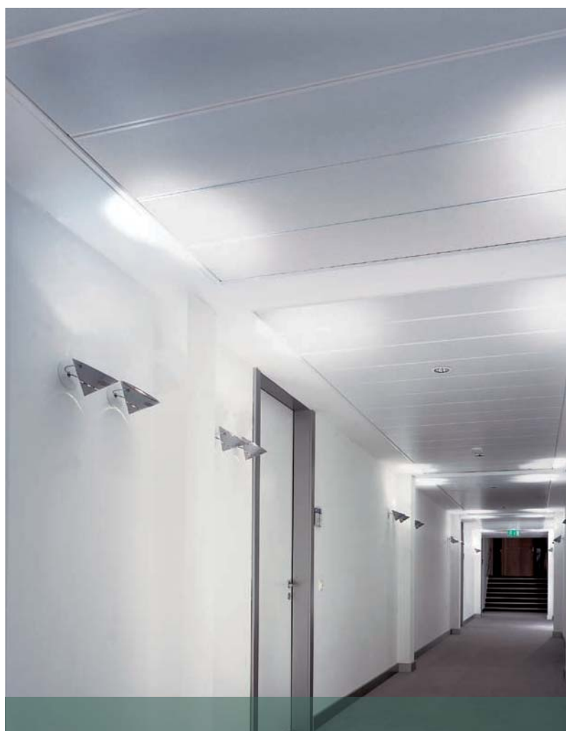
Exposed System F
