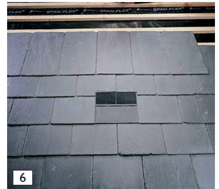
6 At gauges below 225mm, slight trimming of the slates in the course above the vent, may be required.
