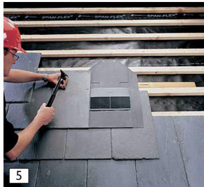
5 When fixing the adjacent 500mm x 250mm slates, they should abut the main vent body (see guide marks on vent).
