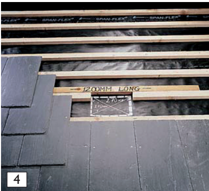
4 Continue to follow the 600mm x 300mm fixing instructions - Steps 3-7 (shown overleaf).
