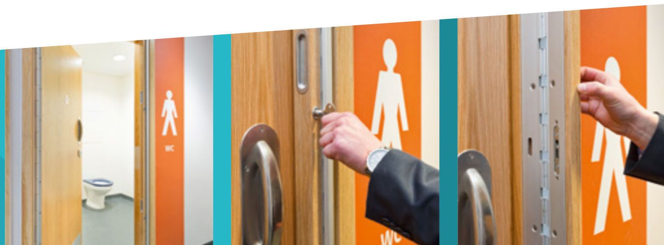
Normal operation the door opens inwards for staff and service users alike.
