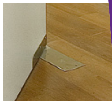
The floor spring box is recessed in to the floor to provide a discrete, anti ligature solution.
