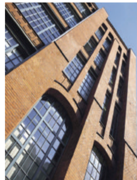
AA ® 720 Renovation "TIP" used on a steel window replacement project
