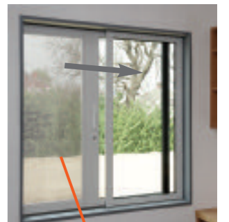
Mesh comes across the window on opening allowing good visibility but preventing the flow of contraband in or out of the window
