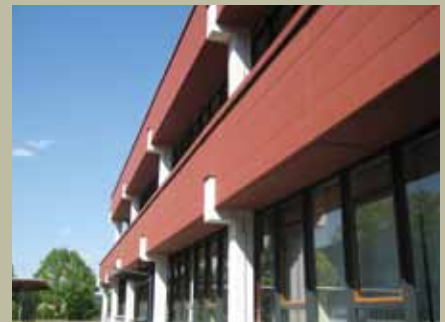
Comprehensive School Battenberg, Germany
