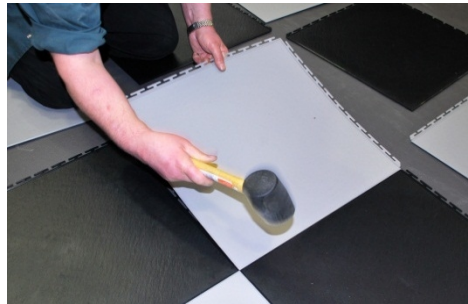
Pic 5. Don't force the tiles, offer up the corner of the tile and gently hammer the joints together.
