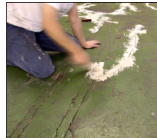
Pic 2. Sweep the floor, remove any highpoints and patch repair or level any cracks or low points.
