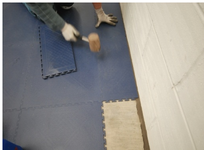
Leave a minimum of a 5mm gap between the tiles and any fixed point (walls and machinery)
