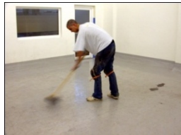
Pic 2. Sweep the floor, remove any highpoints and patch repair or level any cracks or low points.
