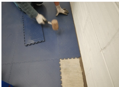
Leave a minimum of a 5mm gap between the tiles and any fixed point (walls and machinery)
