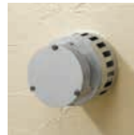
Balanced Flue (No chimney required)
