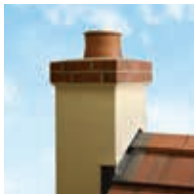
Brick or Stone Chimney (Class 1)
