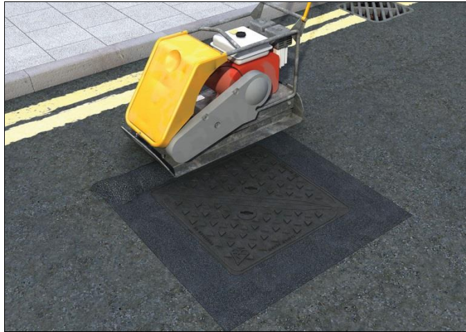
Figure 8 Final compaction of Ultracrete Instant Road Repair
