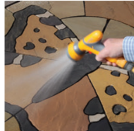
1. The paving is soaked with a hose. It is impossible to over-water the paving and joints.
