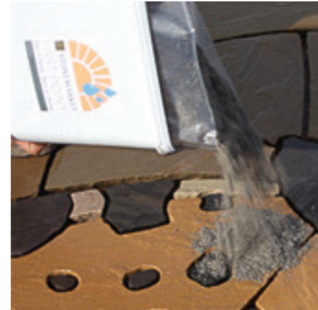
3. The Fast Point material is poured onto the paving
