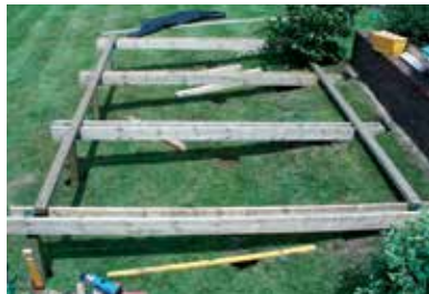
....building the support beams....
