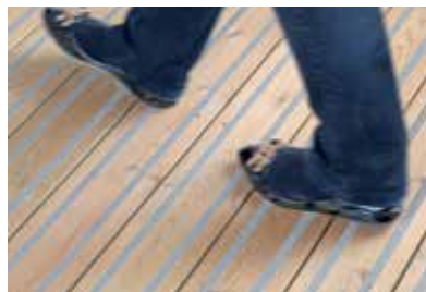
Fig (i) Boards placed at right angles to pedestrian traffic.
