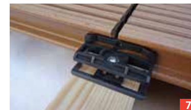
Screw at end, expansion all to right.
