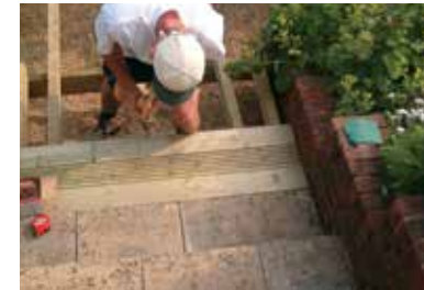
....fixing the first decking boards....
