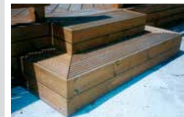
Steps can be created by extending different levels of sub frame.
