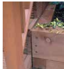
Timber-Tite countersunk versus proud hex head.
