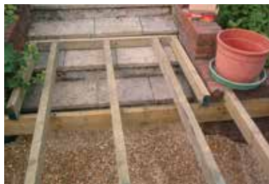
....ledger board fixed to existing steps....
