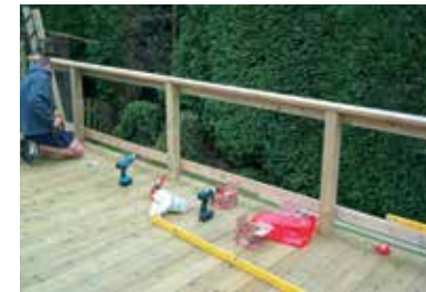
....fixing the handrails and base rails....
