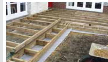
Step frame set on compacted hardcore and weed barrier.
