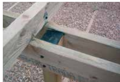
....joist fixed over the beams....
