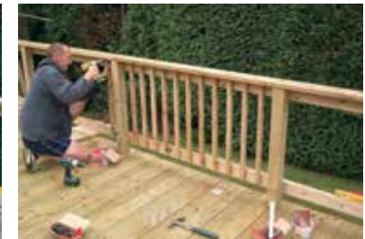
....fixing the balustrades....
