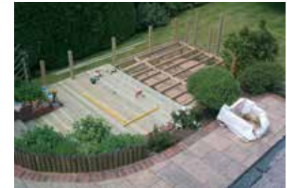
....fixing the decking boards throughout the deck....
