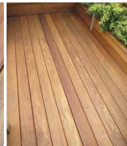
Q-Deck Garapa hardwood - cleaned and re-treated with Deks Olje D1 Pro® (Honey Tinted).
