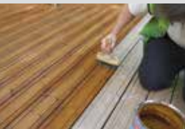
Weathered and cleaned Q-Deck Lunawood® finished with Aquadecks® Teak.
