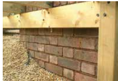
....ledger board fixed to existing wall....
