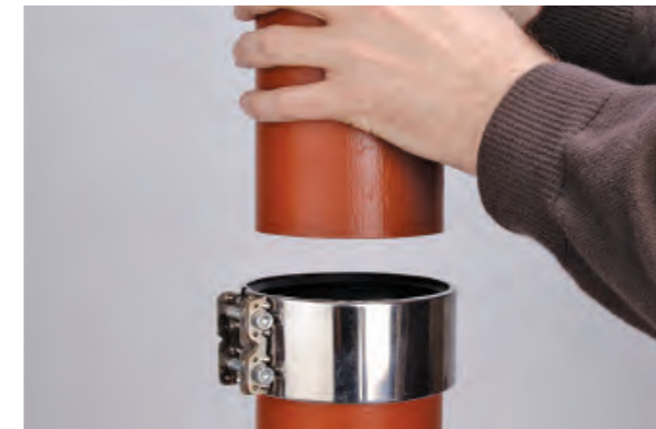
3. Ease the next pipe or fitting into the coupling as step 2.
