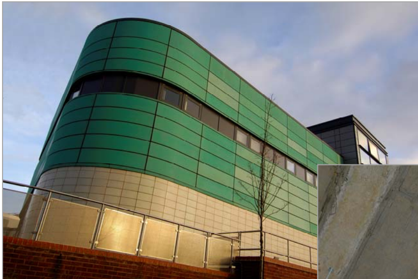
Derby Hospital Installed by East Goscote Plumbers Completed with Skanska
