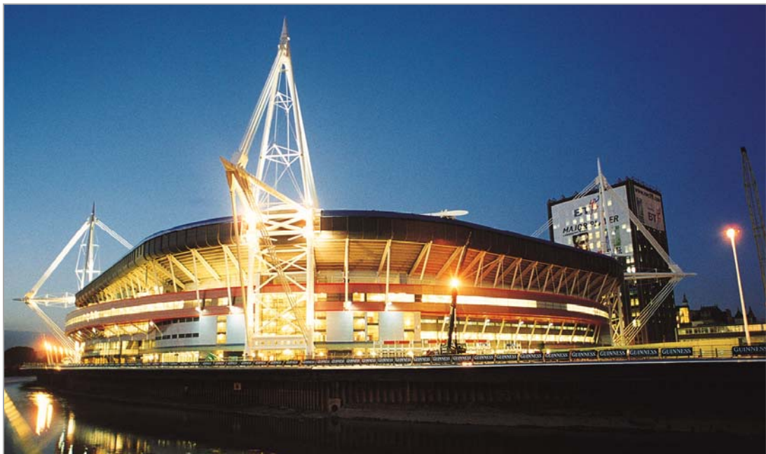
Millennium Stadium Installed by Drake & Scull (Emcor)
