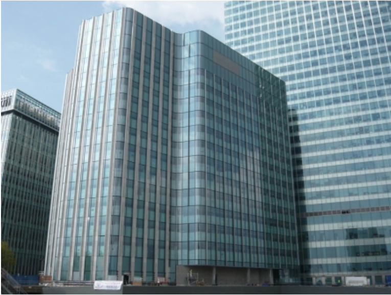
Canary Wharf BP2 Completed with Aquasafe Environmental
