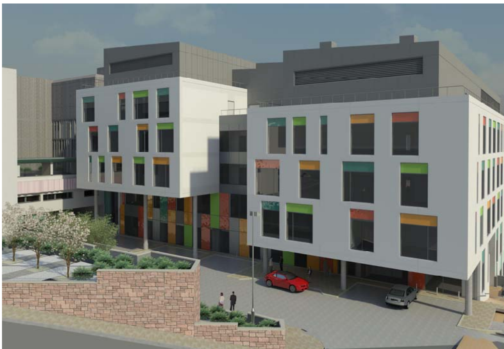
BRI, Bristol Royal Infirmary Installed by Crown House Technologies
