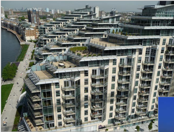
Battersea Reach Consultant White Young Green Installed by Dennis Cox
