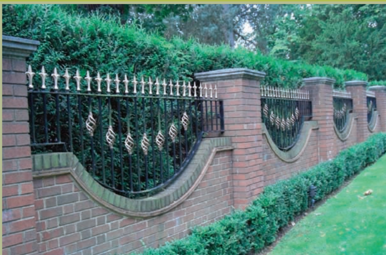
Decorative Railings, that were manufactured to match a pair of gates, a basic railing design with finials on top and twist scrolls in the centres.
