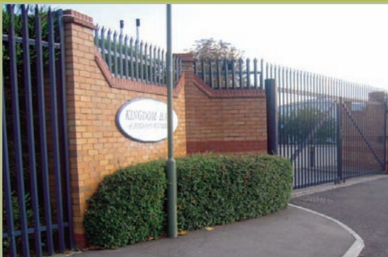
Palisade fencing with manual gates to match, lockable by key.
