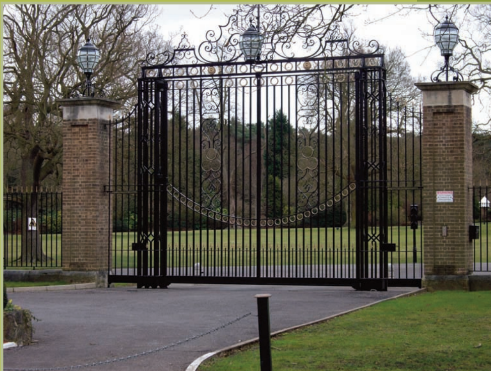
Large sliding gate with decorative infill, access control and traffic light system with ornate support posts and top arch. Gates were a bespoke design
