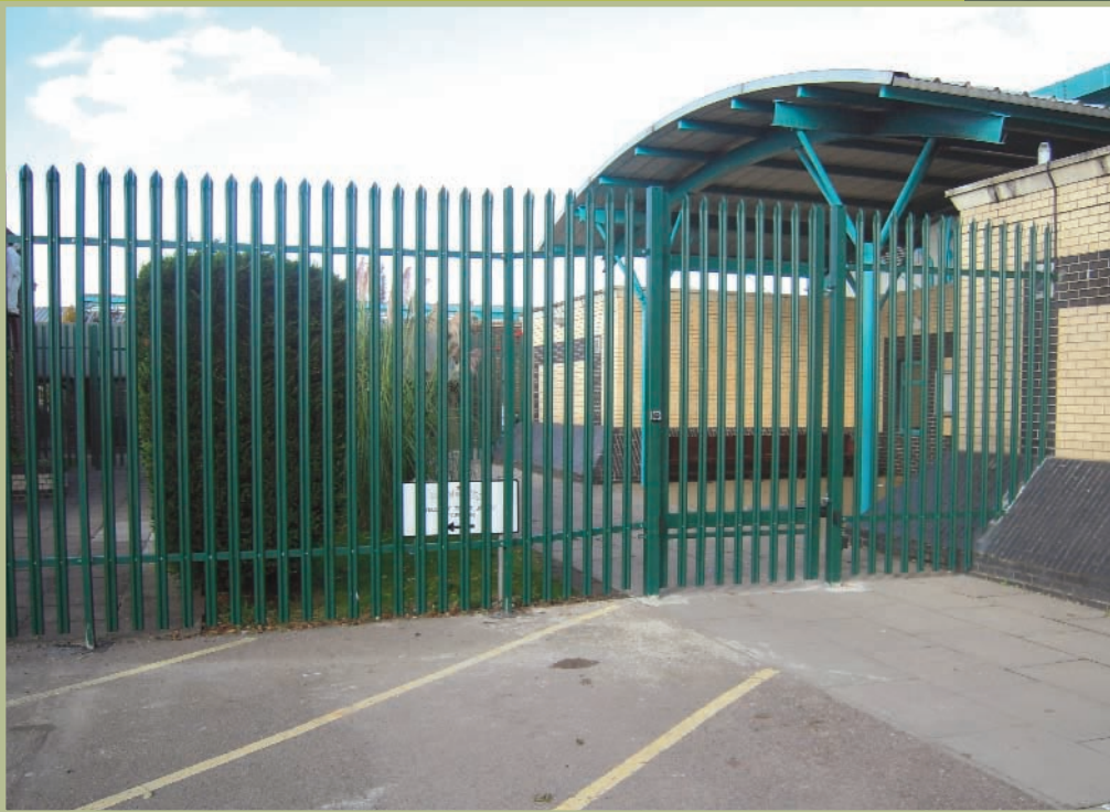
Pallisade pedestrian gate automated with access control and a hydraulic ram operator
