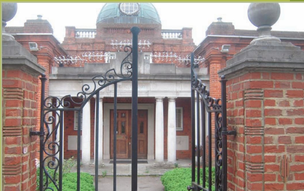
Anti Climb Spikes and Steel gate
