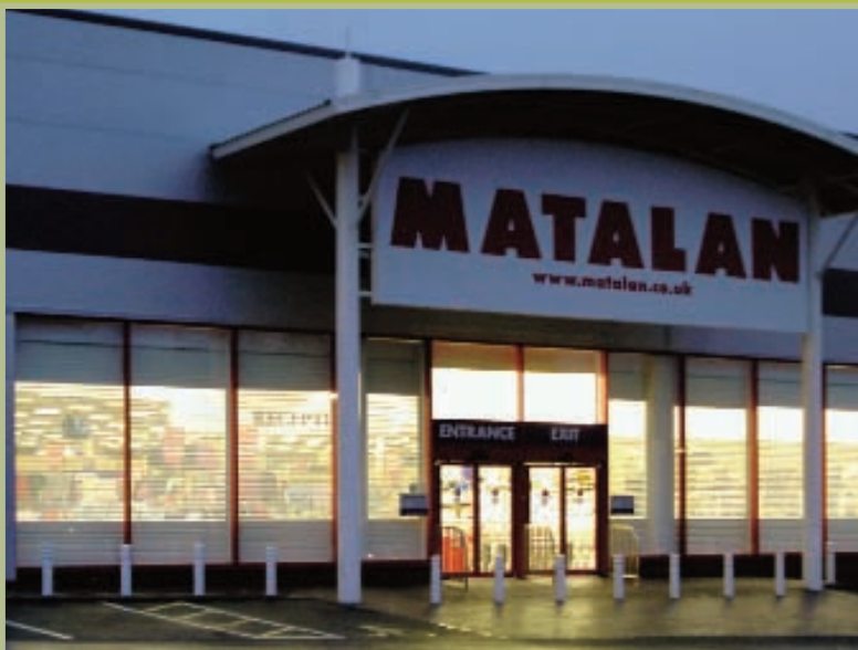
HS75 steel shutters incorporating perforated and solid lath sections. Shutters are operated by group control.
