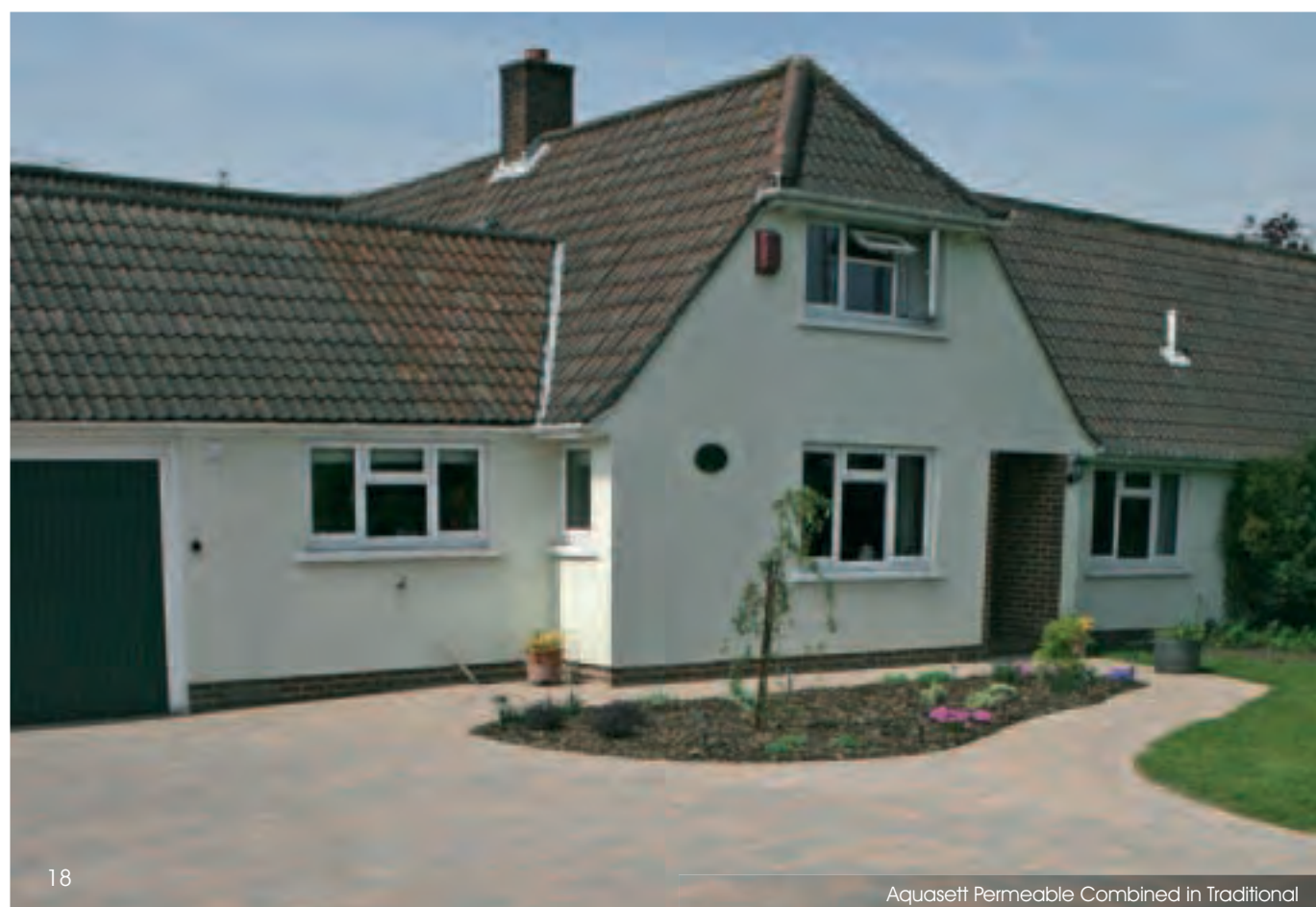
Aquasett Permeable Combined in Traditional
