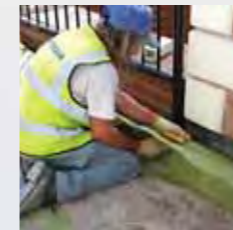
7 Trim Inbitex geotextile to finished paving level
