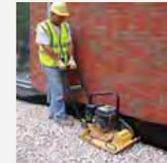
6 Compact for laying course
