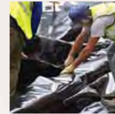
1 Fitting welded membrane
