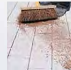
9 Finally brush in the 2-4mm grit surface dressing
