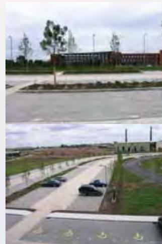
6,500m 2 of Aquaflow ThermaPave geothermal system supplying 580kW of heating and 200kW of cooling to the 2,700m 2 office building
