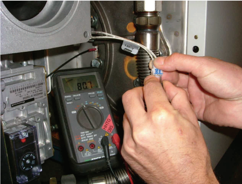
Figure 7.2.3 - Hot Surface Ignitor Check 150c/ 200c/ 250c
