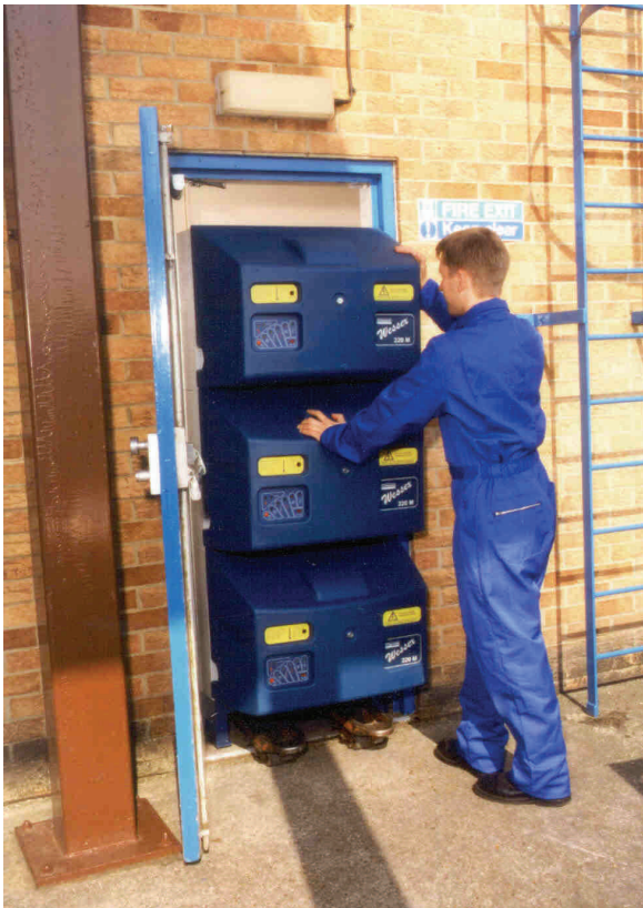
Figure 2.2 - Boiler Positioning
