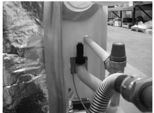
Figure 9.2 - Water Flow Switch
