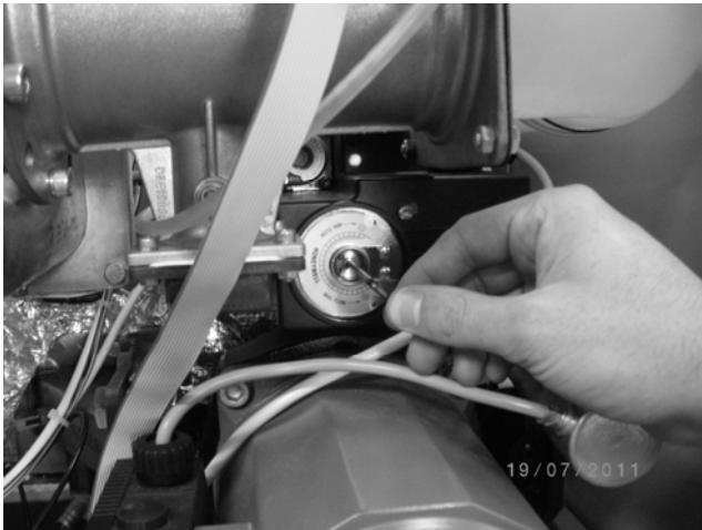
Figure 7.6.1- Adjusting gas valve throttle
