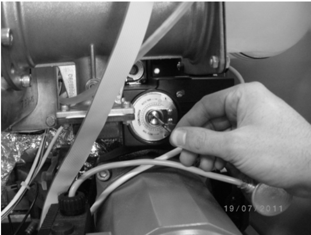
Figure 7.6.1- Adjusting gas valve throttle
