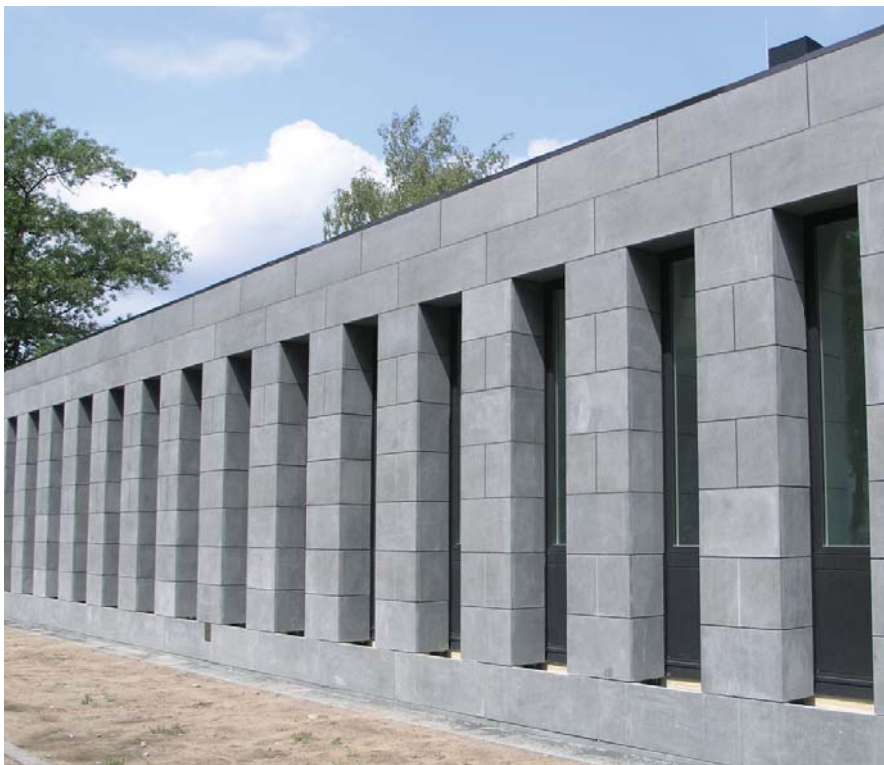
Police station in Eberswalde, Germany
