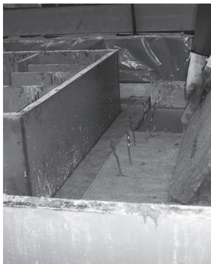
Installation at the precast plant: SPA-A
