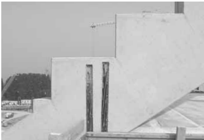
Connection; grandstand in stadium – supporting element
