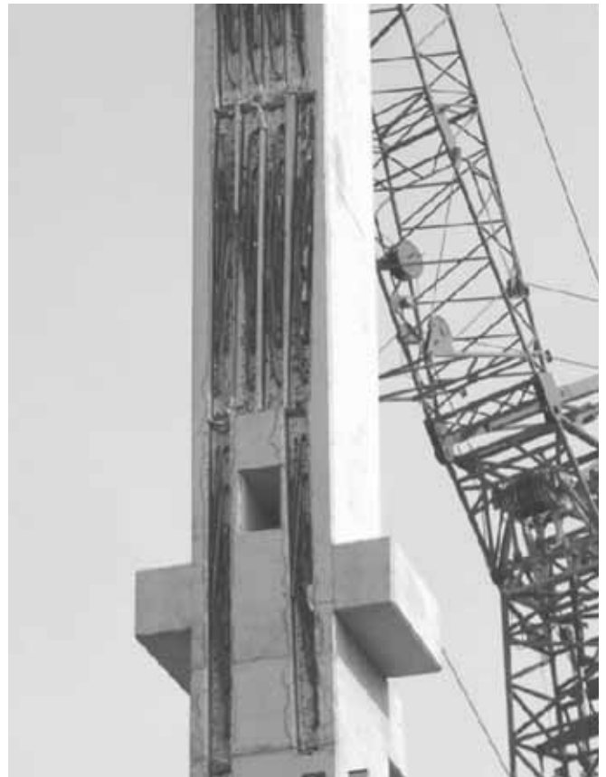
Connection; column – wall
