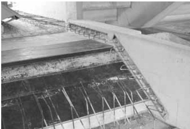
Connection; wall – stair landing
