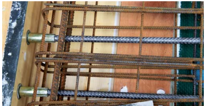
INSTALLATION OF FIXING ANCHORS
