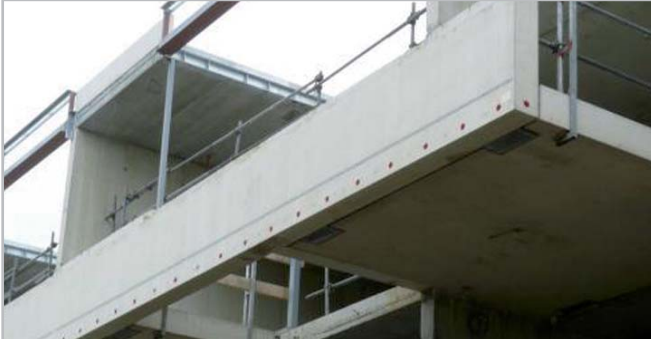
FIXING OF BALCONY RAILINGS
