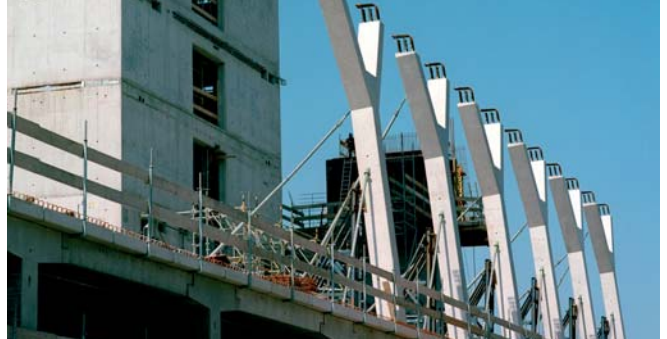
FIXING AND ADJUSTING PRECAST ELEMENTS
