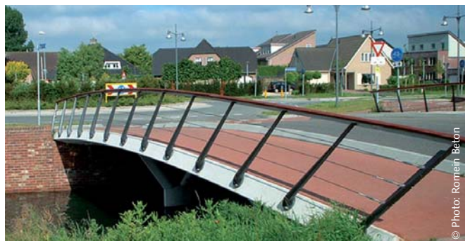
FIXING OF BRIDGE RAILINGS
