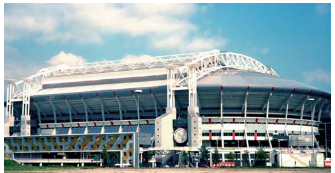
APPLICATION IN PRECAST ELEMENTS FOR STADIUMS
