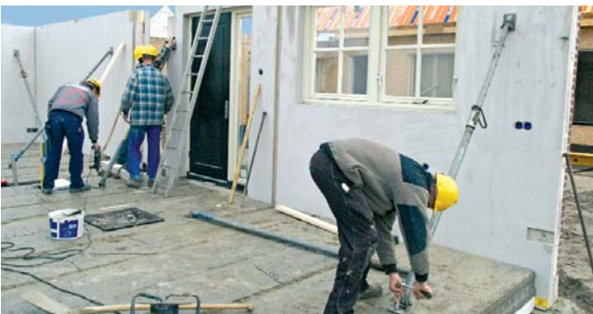
FIXING OF PROPS ON PRECAST ELEMENTS
