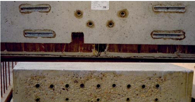
CAST-IN FIXING ANCHORS
