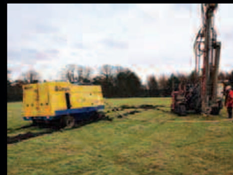
Siting a drilling rig - without Ground-Guards!
