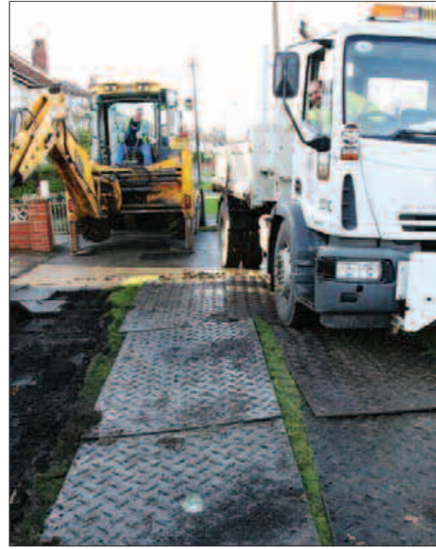
Ground-Guards RoadTrack panels provide verge protection for highway maintenance works.
