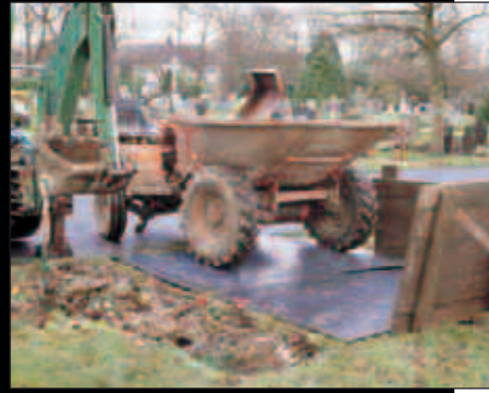
Smooth topped boards enable soil to be easily shovelled back into the grave.
