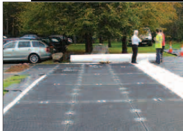
Monitoring the progress of a temporary car park installation.
