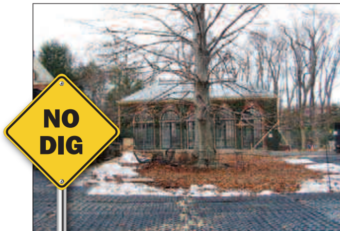
Ground-Guards in use for protecting tree roots from construction site damage.
