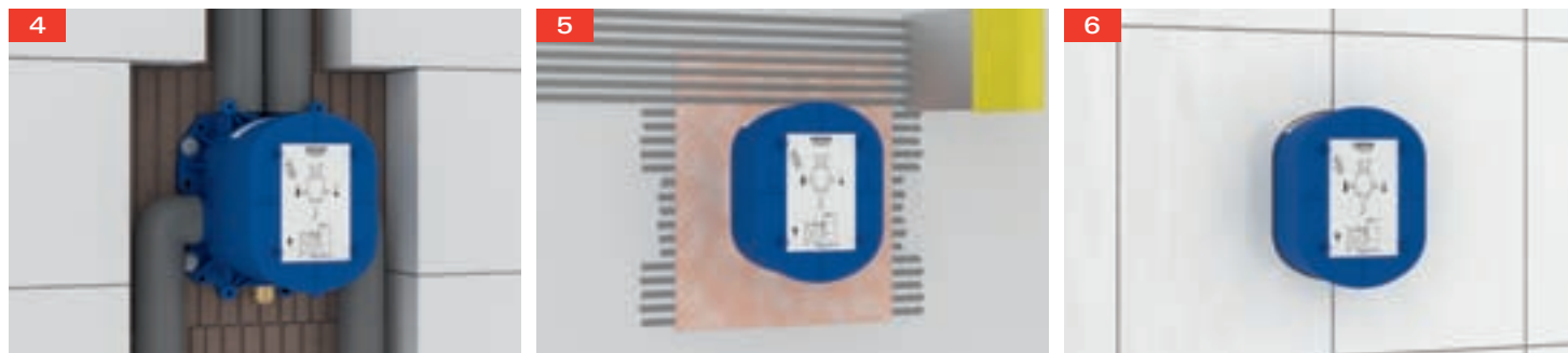
4 Make good wall recess Note markings indicating the correct installation depth
