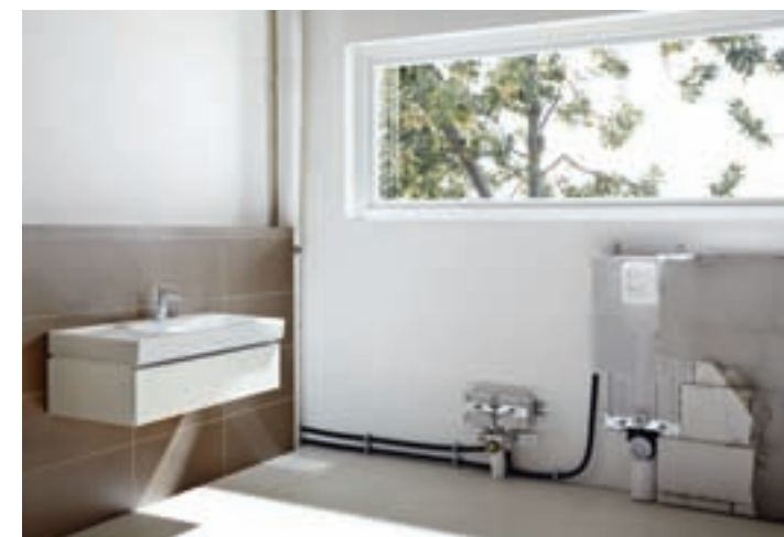
Walling in, plastering, tiling
