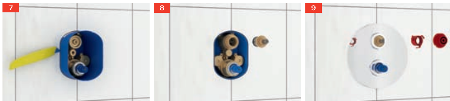
7 Remove protective cover Cut fitting box so it is flush with the tiles
