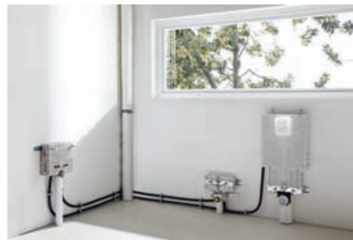
Roughing-in installation
