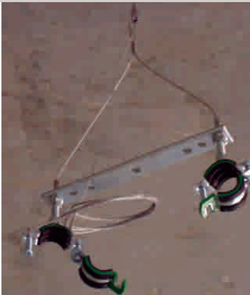
1. Fix using wire anchor, eyelet anchor or M6/M8 adaptor into concrete.
