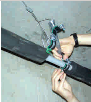
2. Attach pipe clamps to M8 studs.
