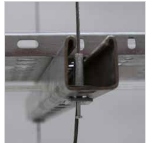
Step 3 - Pass the wire rope through the Trapeze and adjust the height.
