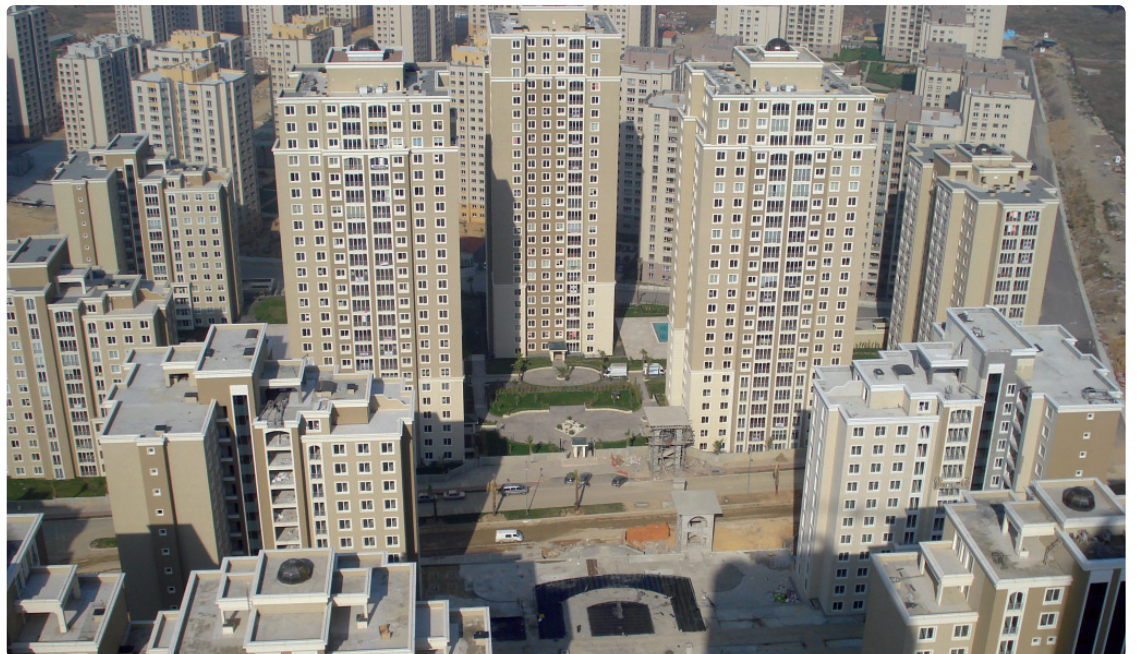
Figure 5: A total of 11,945 window surrounds, each using approximately 4m 2 of GRC, plus 15,898 decorative elements on 1742 flats in Istanbul.
