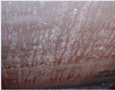
Vapour permeable underlay (type LR) with smooth underside showing condensate run-off and dripping
