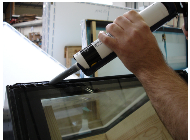
Figure 6 - Applying polyethylene expanded foam-backing rod and silicone.
