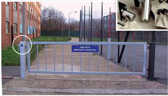
The communal parking area at Nelson Mandela House
