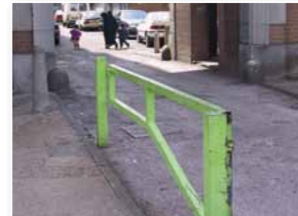
Gates left or pinned open will not prevent unauthorised access
