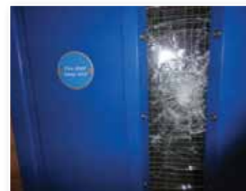
Axe attack on the anti-vandal 3tiervision™ panel. The fire door is still able to function with no breach to the inner section of fire resistant glazing.
