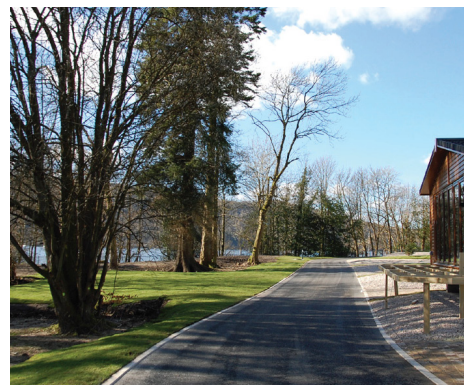
Fallbarrow Park, Windermere: Completed CellWeb TRP® Installation
