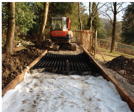
Fallbarrow Park, Windermere: CellWeb TRP® Installation
