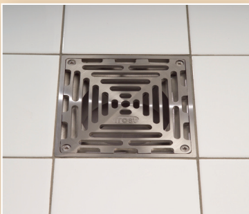
Stainless steel grating in a tiled floor
