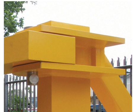
Locking Pin securing crash beam into closed position
