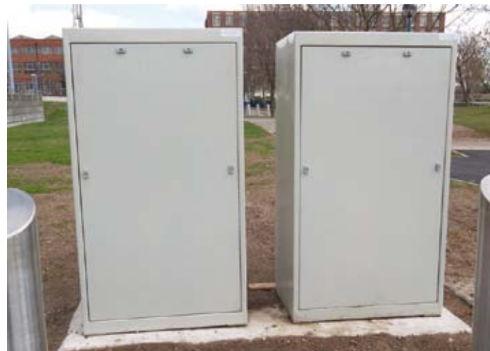
Hydraulic control cabinets for Terra Blockers and Active Terra Bollards are recommended to be installed within 10 metres of the unit, within site in a secure location.
