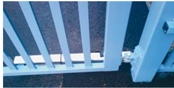
Locking Pin securing gate leaves into closed position
