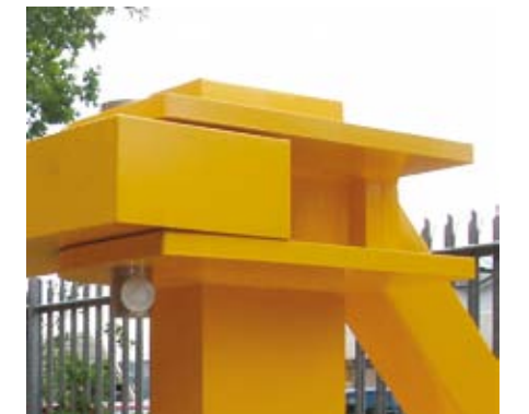
Locking Pin securing crash beam into closed position
